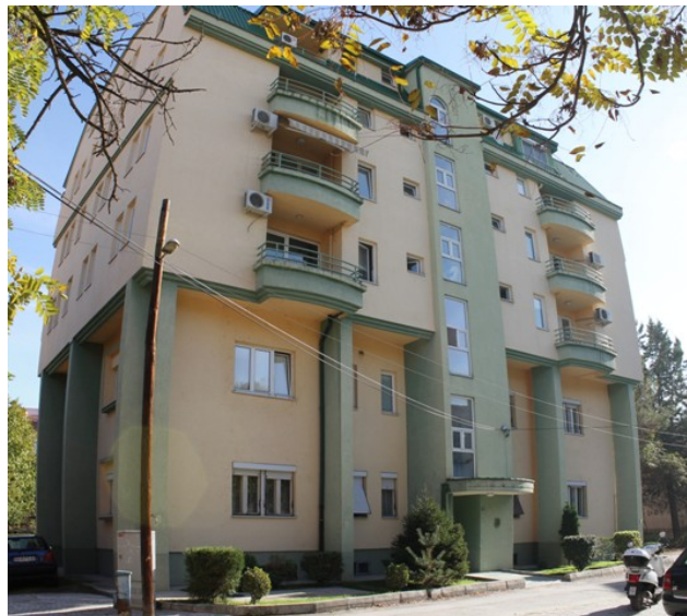
Example of a two storey building that was ‘upgraded’ with an additional four floors
